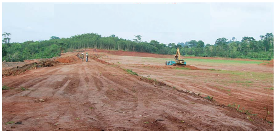
Preparation of the tailings dam to be re-utilised at Konongo.
